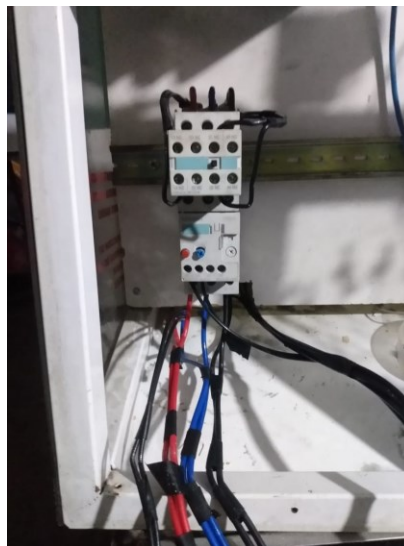
Figura 4-36: Contactor de 40 amperios
